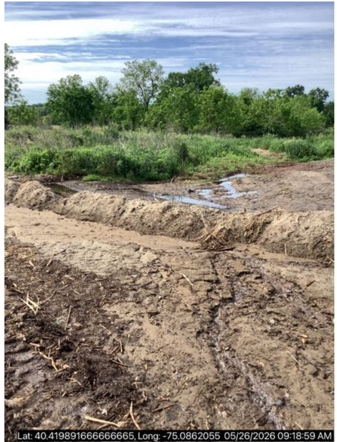
Photo #6 Regraded area.
