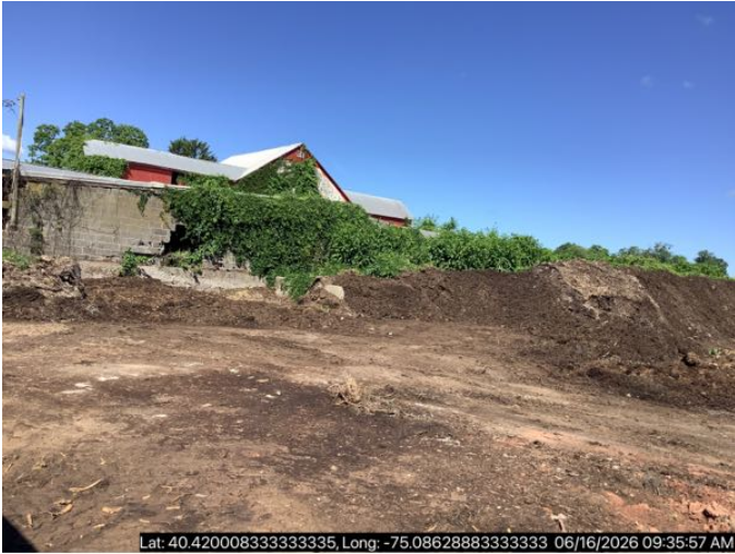
Photo #5 Oldest windrow compost pile and regraded area next to barn.
